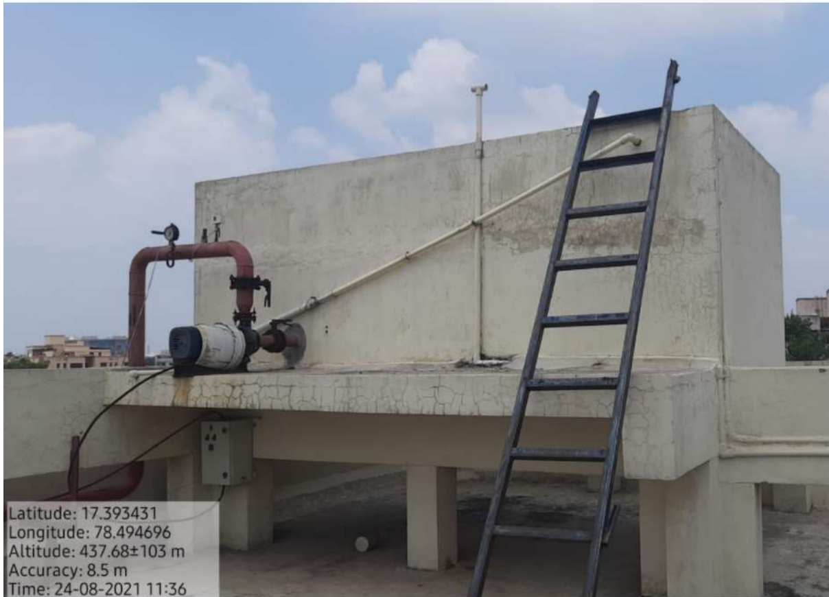
Construction of tanks and bunds
