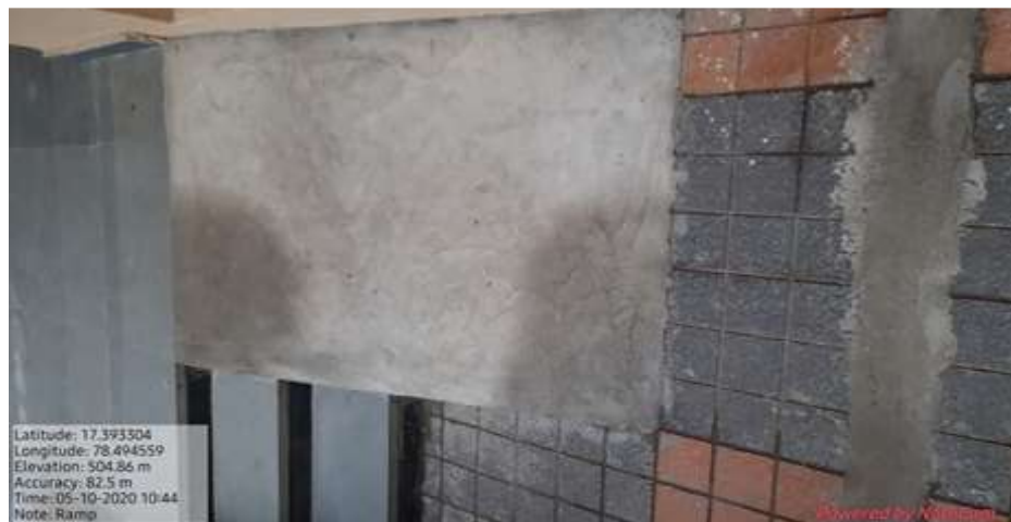
Disabled Friendly ramp
